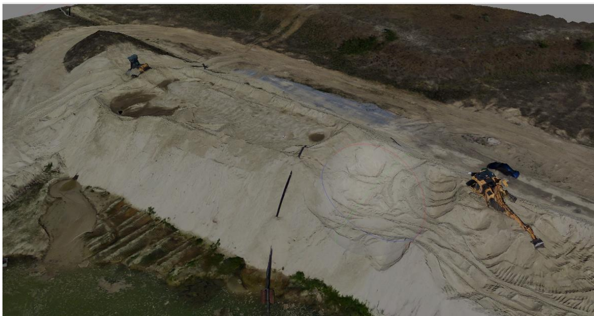
Figure 5. Initial three-dimensional model of the warehouse surface based on the results of quadcopter surveying.
