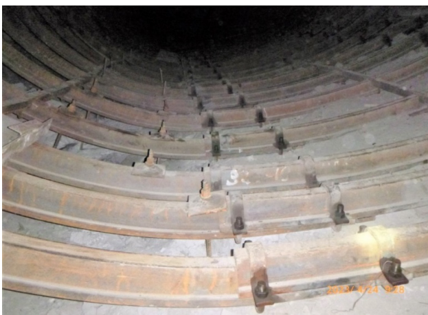
Fig. 12. Horseshoe-shaped reverse vault and anchors before concreting
